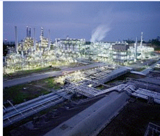
GTL plant Processing
